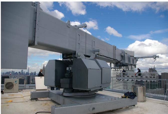
BMU - Fixed position with slewing turret, telescopic boom retracted
