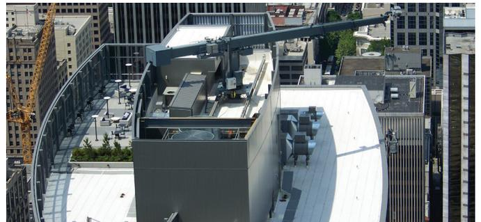
BMU - telescopic mast raised, telescopic boom deployed
